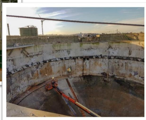
**The solution:** Initial works consisted of various surveys and tests to determine the scope of remedial works required, including structural surveys, carbonation tests and chloride profiling. Upon completion of testing, internal concrete defects located on both tanks were identified, broken out and repaired using a high strength, polymer modified SikaMonotop 612 repair mortar, complete with the provision of protective coatings.
